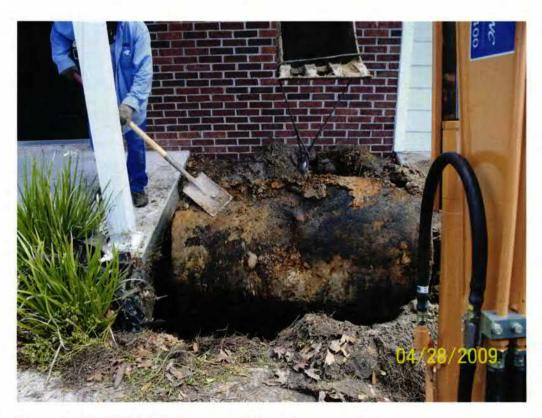
Picture 2: UST 289Birch being removed from the excavation.
